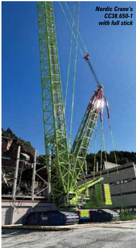
Nordic Crane's CC38.650-1 fully rigged
