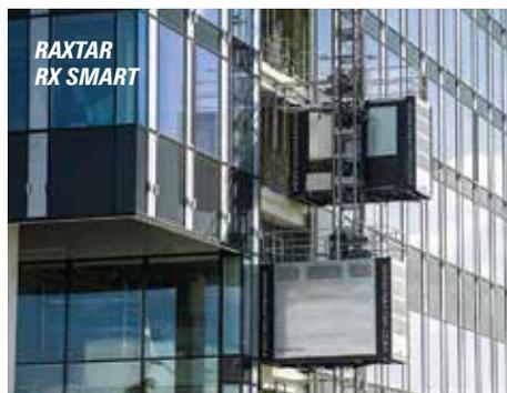
hoist with a payload of 2,300kg and lift speed of 36 metres a minute. Other features include quiet operation, standard C-gate and programmable landings with hoist calling system.
