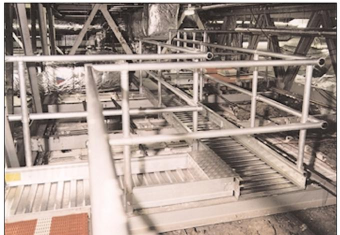
Aluminium walkways from UpRight UK Special Products have played a critical part in a £3.5 million contract by Mansell for client BAA to upgrade fire safety, roof void access and services at Heathrow Terminal 1.
