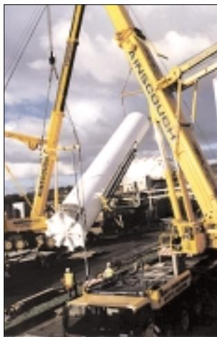
The Group's National Heavy Crane Division provided an 800 tonne AC2000 Demag as the main crane for the lift and also one of its 400 tonne Liebherr's for the tailing operation.
