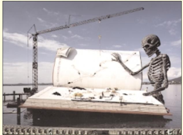
**Opera with Liebherr:** A pontoon-mounted Liebherr tower crane has played a dramatic role in dismantling a large floating opera stage set in Bregenz, Austria. The Liebherr 71 K was used to remove the 25 metre high book and the skull of a skeleton which weighed 3.6 tonnes.
