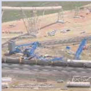
The Lampson Translift and its fallen load
