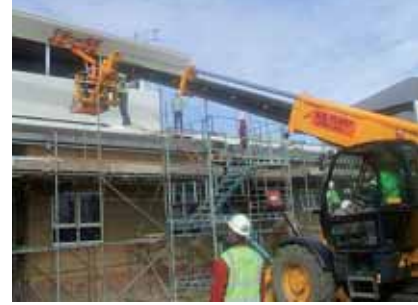
An Oktopus suction device fitted to a telehandler.
