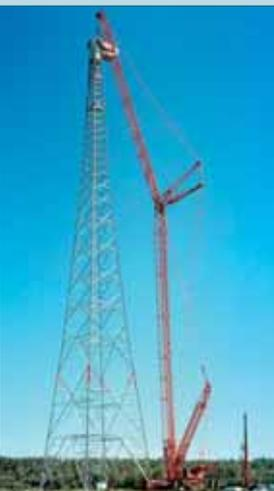
**A 750 tonne Liebherr LG 1750** lattice boom mobile crane erects the world's tallest wind turbine near Cottbus, Germany. The windmill has a 160 metre hub height and blade tip height of 205 metres.
