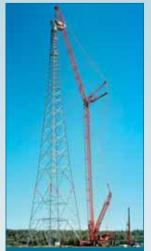
A 750 tonne Liebherr LG 1750 lattice boom mobile crane erects the world's tallest wind turbine near Cottbus, Germany. The windmill has a 160 metre hub height and blade tip height of 205 metres.
