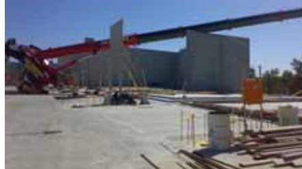
The crane tipped and the boom came to rest on a panel
