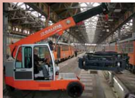
A crane goes straight to work lifting a heavy undercarriage into place.
