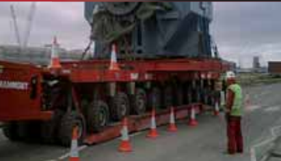
After the equipment was unloaded it was moved to its foundations using SPMT's.
