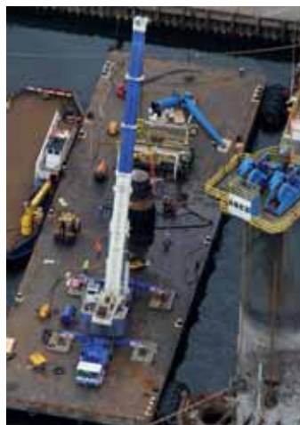
The Liebherr was placed on a barge to get in close to the thrusters.
