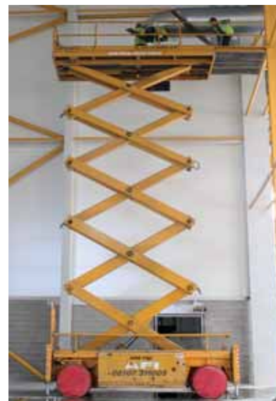
A Liftlux installing ducting.
