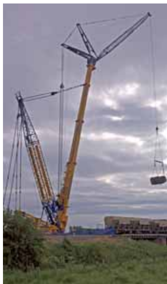
Due to the marshy fenland location and the extensive damage to the bridge, client Network Rail had to build a 1.3km temporary road so the crane could gain access to perform the lifts.
