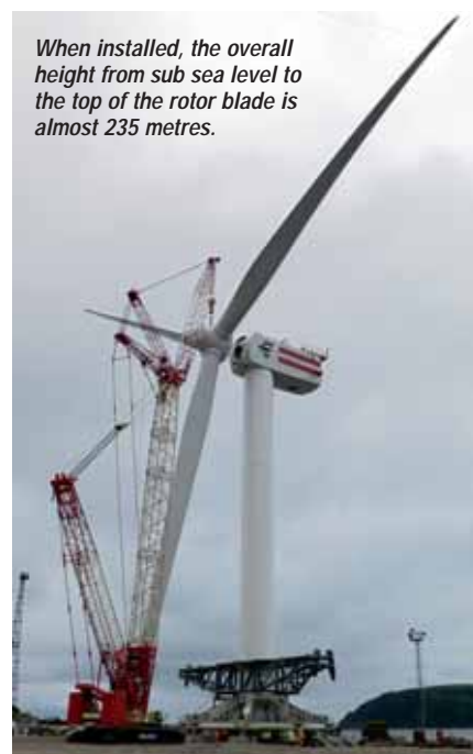
600 tonne skid shoes and 64 tonne push/pull cylinders were used to move the structure up to 89 metres.
