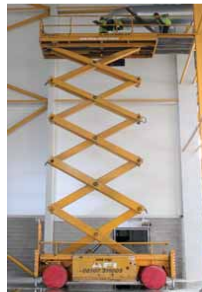
A Liftlux installing ducting.
