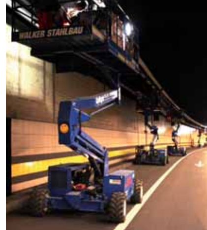
One of the Speed Level's most popular applications has been in tunnel construction and maintenance.
