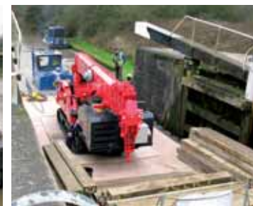
The Unic URW706 moves into place on a pontoon
