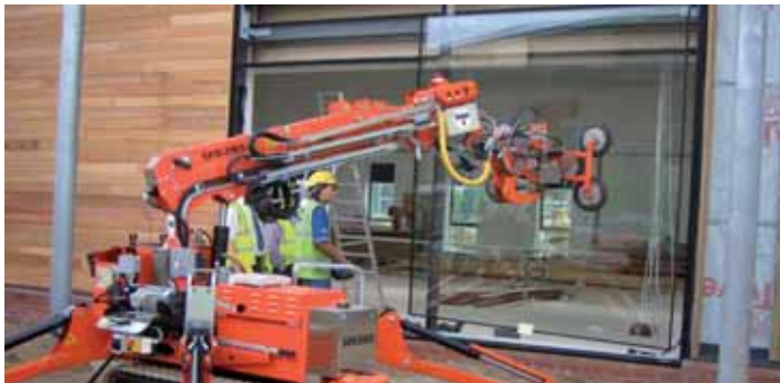
2. Slews around ..... 3. And pops it into position
