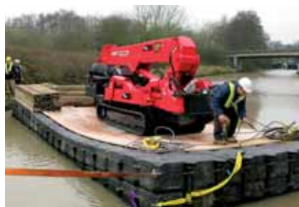
Using the pontoon reduces damage and subsidence to the tow path
