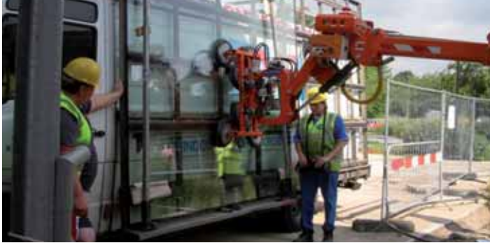
1. The Jekko removes the glass panel from the van
