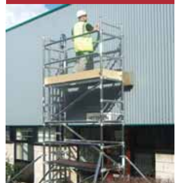
Access tower by Euro Towers Ltd, Northampton
