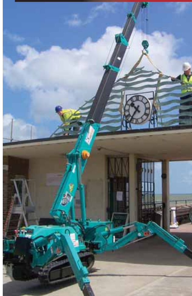
A Jekko machine on glass handling duties
