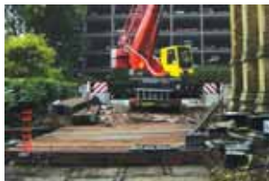
Heavy duty crane access mats
