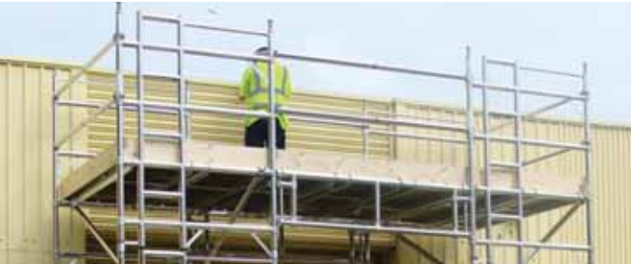
Bridging two towers can not only leave a clear passage underneath, but also provide a larger platform
