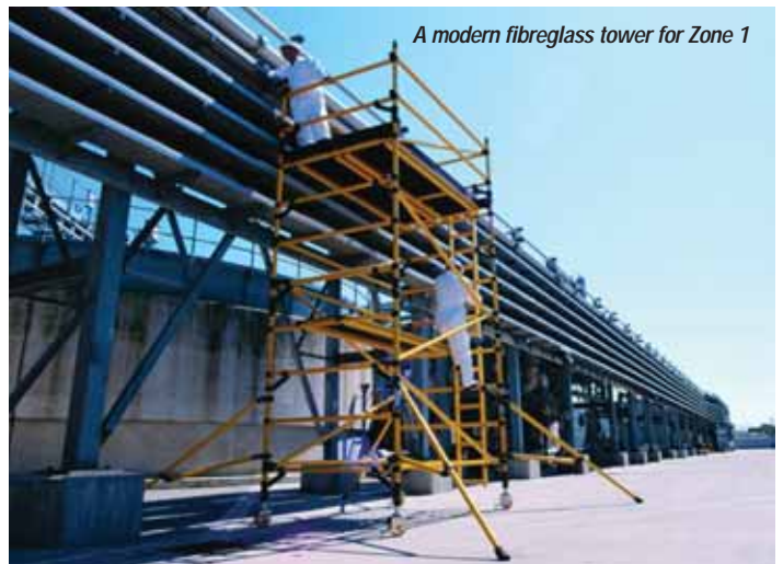
A narrow tower is ideal for confined areas
