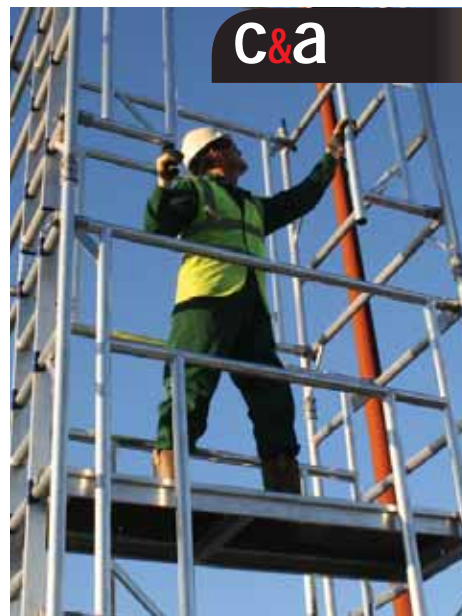
Advanced guardrails are fitted from below.
