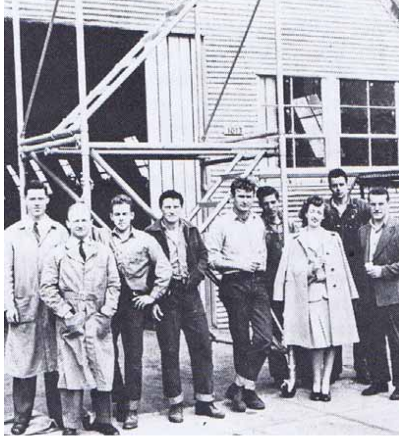
The first production tower - 1947
