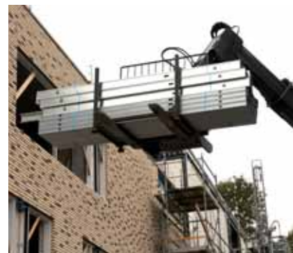
The forks allow a long load to be turned to pass through a restricted opening.
