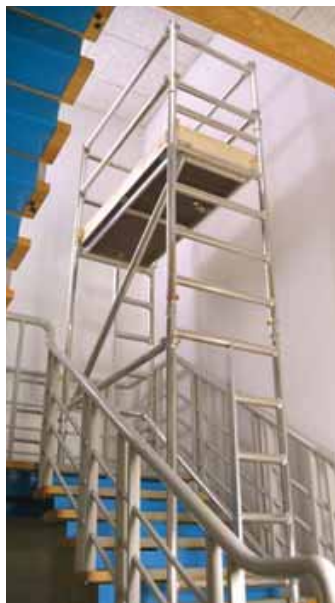
A narrow tower is ideal for confined areas
