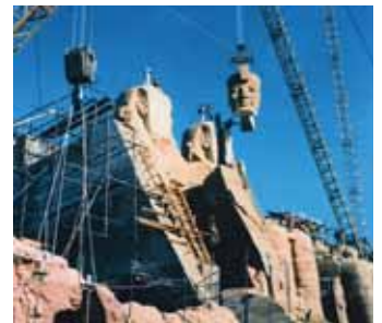
Wolff cranes were involved in the dismantling and reassembling of the two 13th century BC Ramses temples between 1963 and 1968
