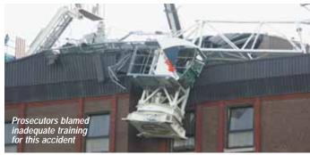
Select admitted breaching health and safety laws while the crane was being climbed, the erectors had failed to secure the superstructure to the tower before trolleying in a new section. The prosecution claimed that they had not been properly
