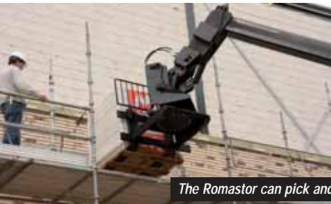
The Romaster can pick and place a load from an angle
