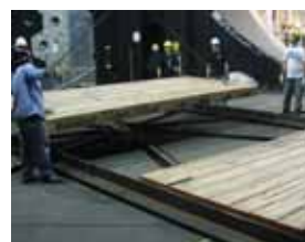
emtek mats manufactured to fit into a specifically designed steel frame
