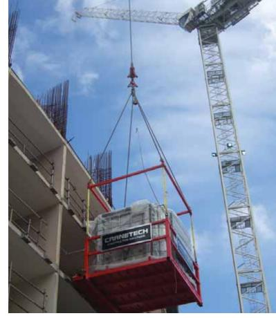
"We quickly realised the potential for the Podlifter as a means of lifting and loading more than just bathroom pods, so incorporated improvements on the original design to make it suitable for plant installation/removal, air handling units, fit out materials etc, in fact anything that is either too heavy or too large to go in a hoist."
