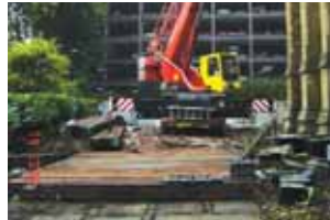
Heavy duty crane access mats
