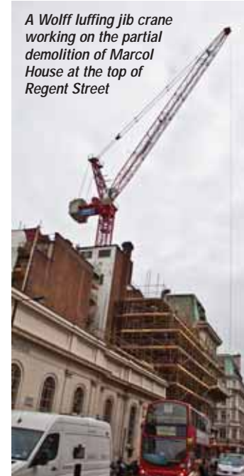
The Wolff 180B luffers are able to get in close to the building's footprint
