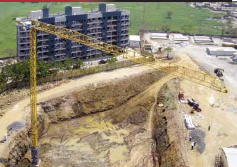
The Liebherr 71EC-B on a custom-built foundation
