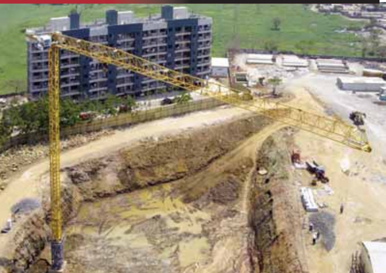
The Liebherr 71EC-B on a custom-built foundation
