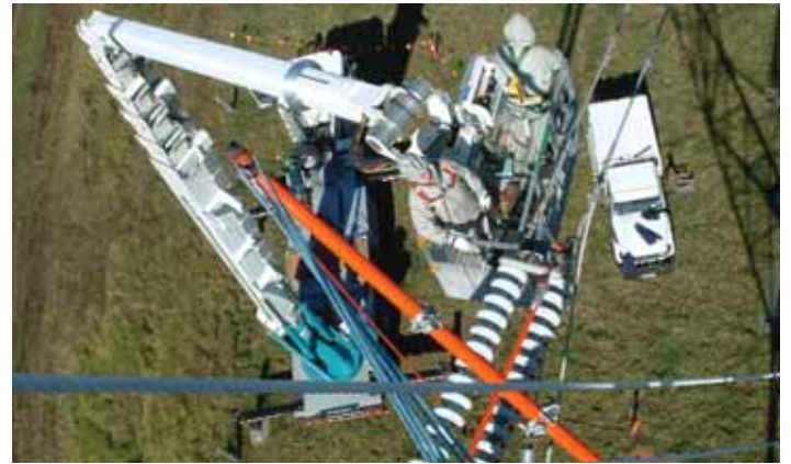
Using the Air-Mat dry cleaning method with a hot-stick applicator
