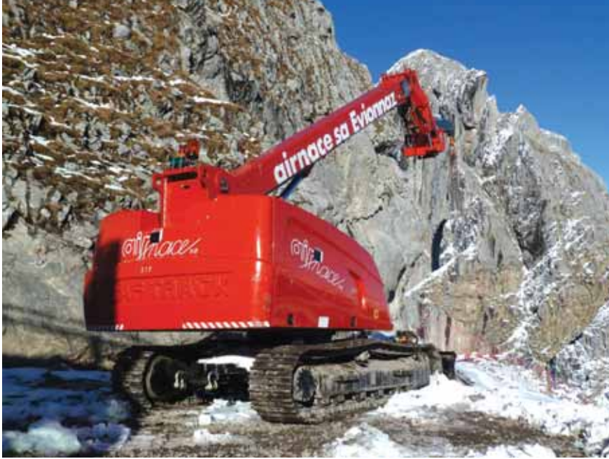
The Giraf Track travelled 10km up exceptionally steep mountain tracks to reach the job site.
