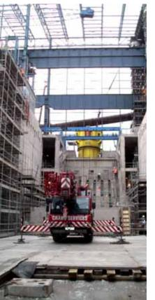
of a platform capable of supporting a 70 tonne crane at the Corus Steelworks in Scunthorpe. Commissioned by Crane Services which was contracted to slab-casters Danieli Davy Distington, the project was initially delayed by six hours due to treacherous winds but was completed after a two-phase installation.
