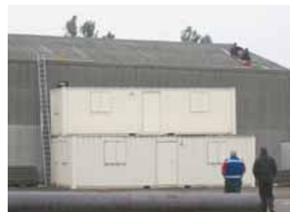
Caught red handed two men working on a roof without suitable equipment
