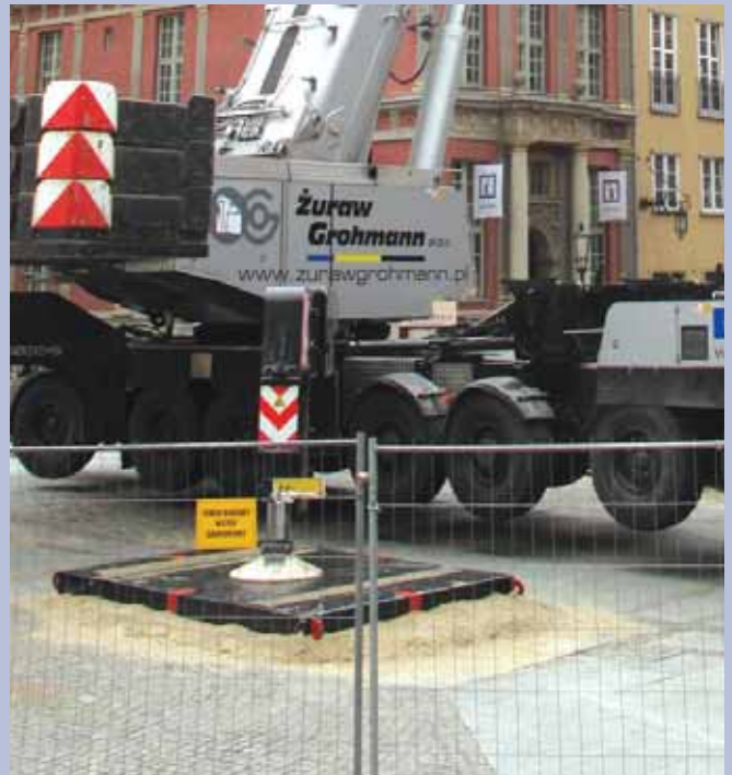
A good example of a steel mat with sand to provide a good base.
