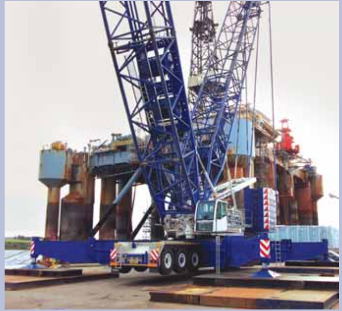
An extensive steel mat set up for a big crane in a dockside application.
