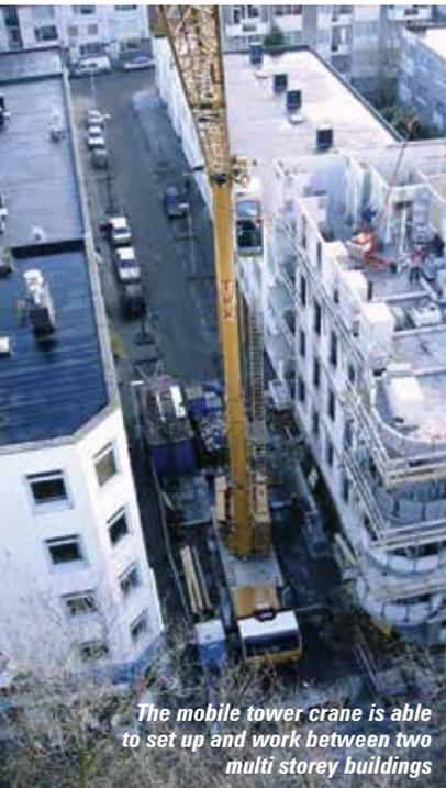
The mobile tower crane is able to set up and work between two multi storey buildings
