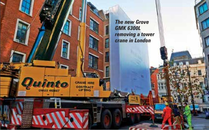
*The new Grove GMK 6300L removing a tower crane in London*
