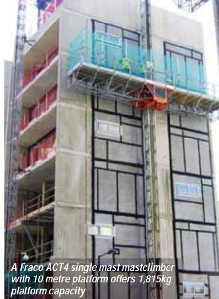
*A Fraco ACT4 single mast mastclimber with 10 metre platform offers 1,815kg platform capacity*
