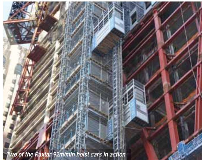
*Two of the Raxtar 92m/min hoist cars in action*
