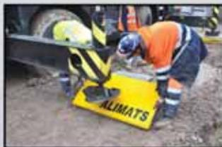
Unique Purpose Designed Modular Interlocking Outrigger Load Spread System
