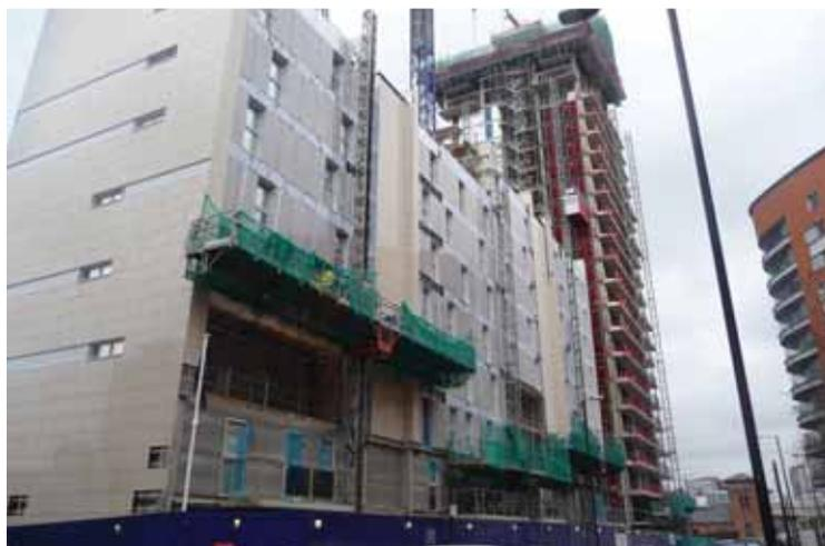
personnel to the upper floors. Perimeter Cuplok scaffolding cantilevered off the 21st and 23rd floors has also been installed to provide access for the roof work. In view of the height and location of Alberta House, Brogan has also erected Combisafe Safety Net Fans as an extra fall protection measure. The nets are designed to catch falling persons, objects and debris protecting both workers and the general public.
