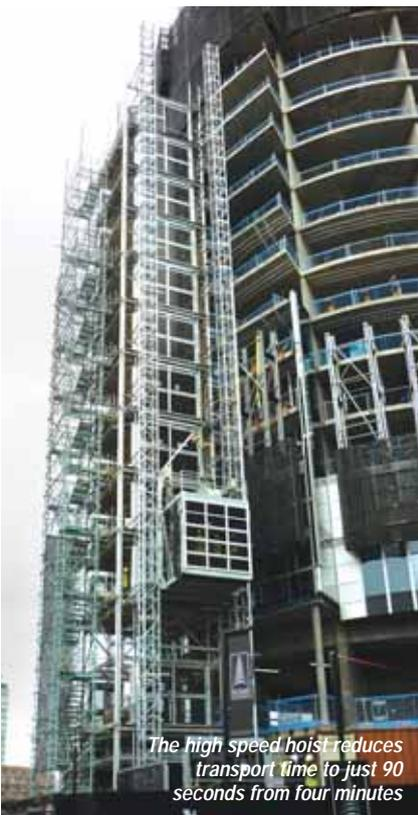
The high speed hoist reduces transport time to just 90 seconds from four minutes
