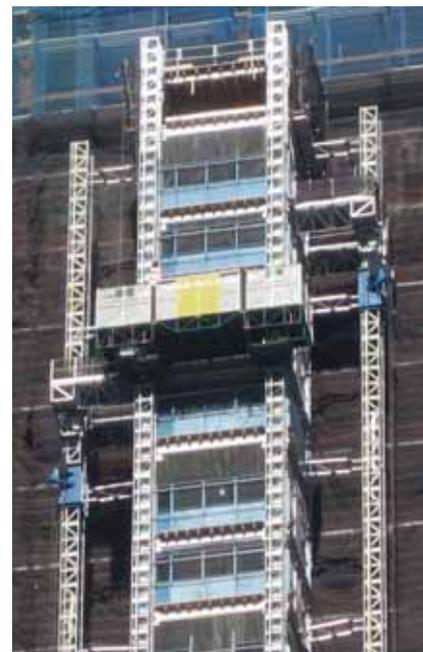
*A Hydro Mobile mast climbing work platform is being used to construct the common tower as it grows with the building.*
