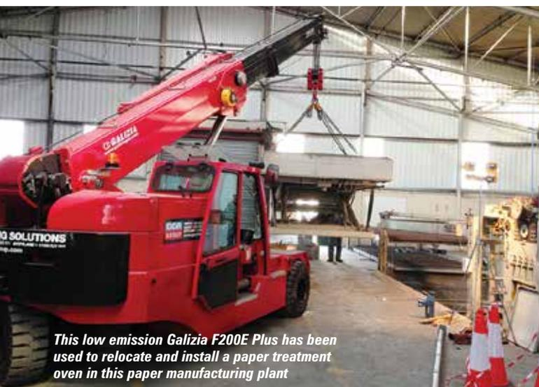
*This low emission Galizia F200E Plus has been used to relocate and install a paper treatment oven in this paper manufacturing plant*
