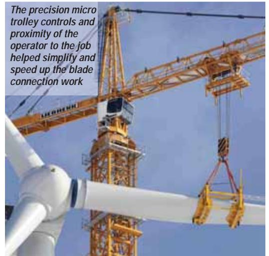
The precision micro trolley controls and proximity of the operator to the job helped simplify and speed up the blade connection work
