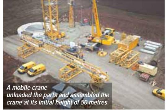
A mobile crane unloaded the parts and assembled the crane at its initial height of 50 metres
