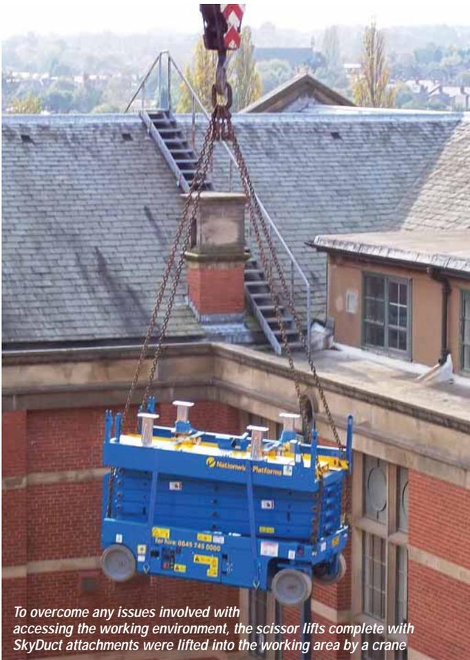
*To overcome any issues involved with accessing the working environment, the scissor lifts complete with SkyDuct attachments were lifted into the working area by a crane*
