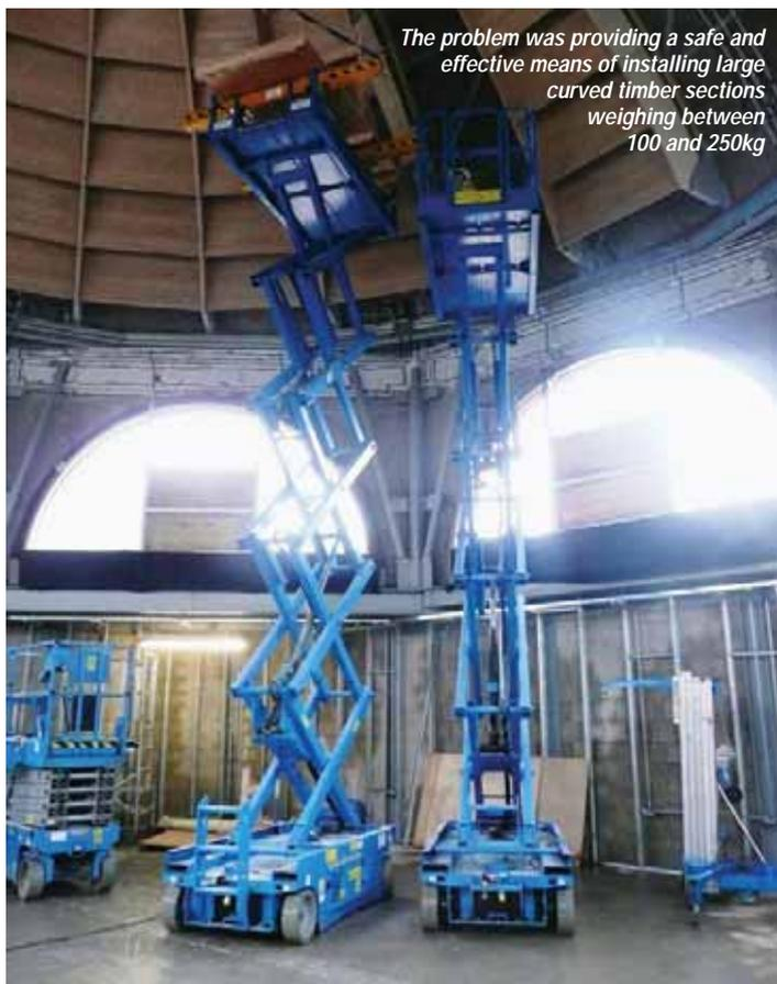
The problem was providing a safe and effective means of installing large curved timber sections weighing between 100 and 250kg
