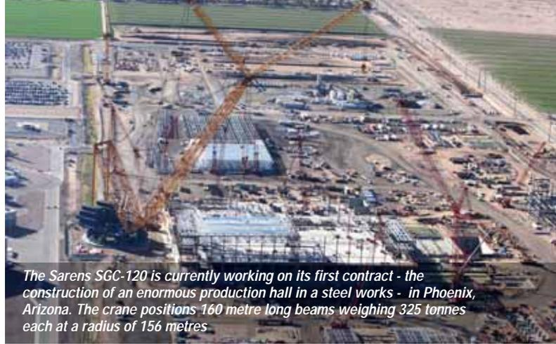
The Sarens SGC-120 is currently working on its first contract - the construction of an enormous production hall in a steel works - in Phoenix, Arizona. The crane positions 160 metre long beams weighing 325 tonnes each at a radius of 156 metres
