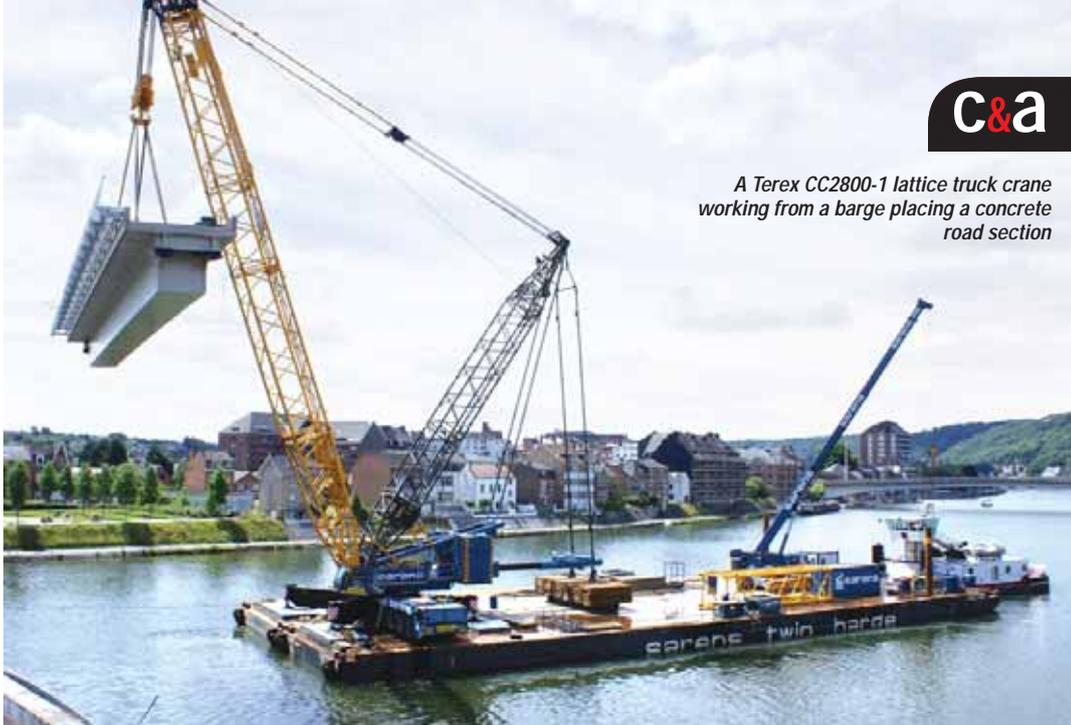
it semi-rigged this can be reduced to one day, but there are associated risks in moving such a crane including not putting down enough load spreading mats, the quality of the access roads which need to be wider and more stable than for trucks etc. There is always a cost factor and corners can be cut to reduce the time or costs," he says.
