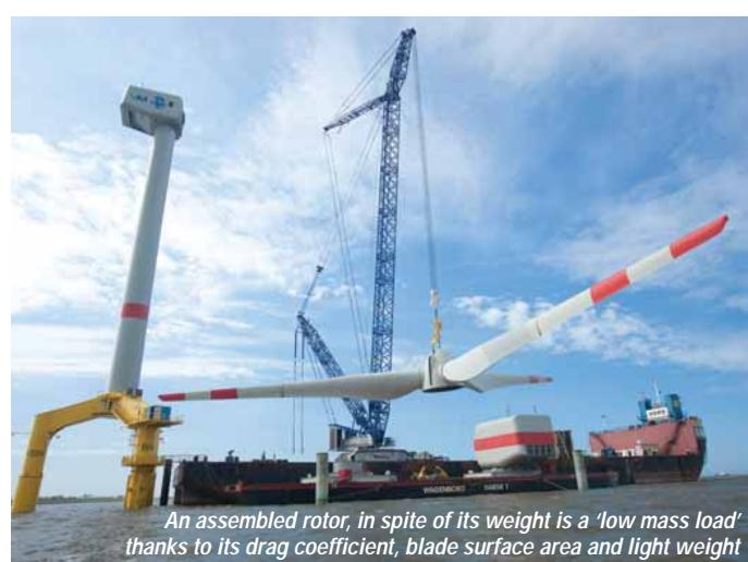
An assembled rotor, in spite of its weight is a 'low mass load' thanks to its drag coefficient, blade surface area and light weight
