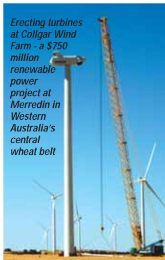
increased number of accidents and have reviewed the wind speed conditions for its equipment when erecting wind turbines. Maximum wind speed should be based on the exposed wind surface of one tonne metre for one metre square or area.
