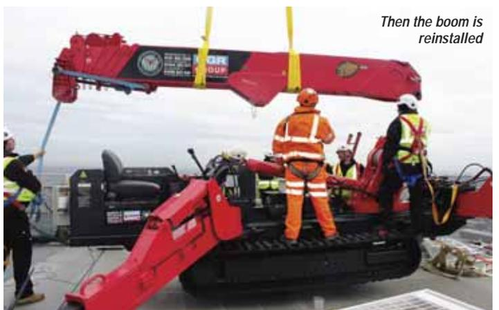
*Working from its 283 metre eyrie the Unic URW706 will lift and place the glass cladding panels from the 62nd floor up*
