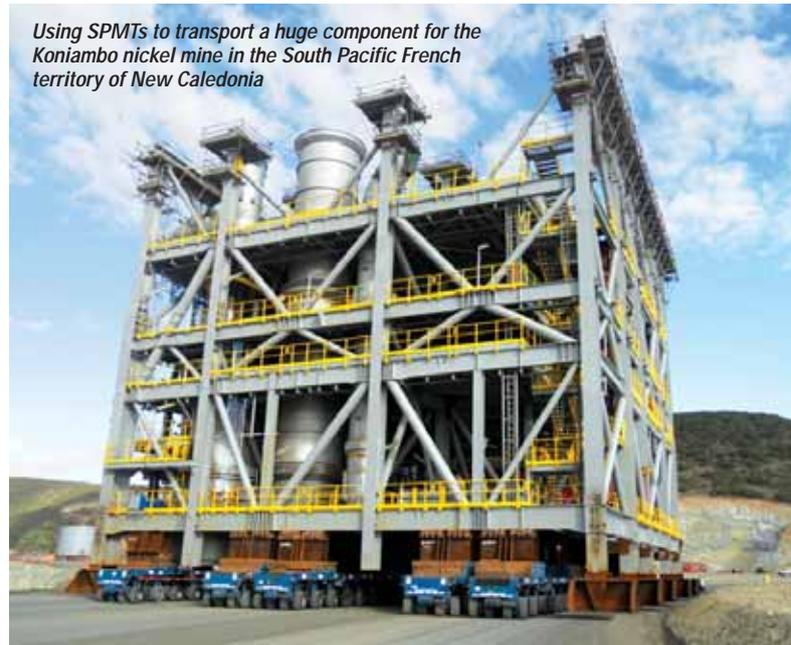
Using SPMTs to transport a huge component for the Koniambo nickel mine in the South Pacific French territory of New Caledonia
