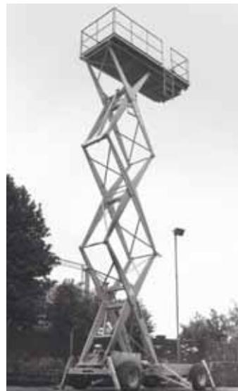
The Manlift SM42RT (above) and the SM31RT were perfect for rental - reliable, easy to use and transport and cheap and easy to repair.
