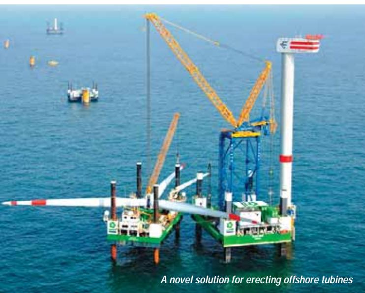
As a general rule, if the crane has an 11 tonne capacity, the wind surface of the item being lifted should be no more than 11 square metres.
