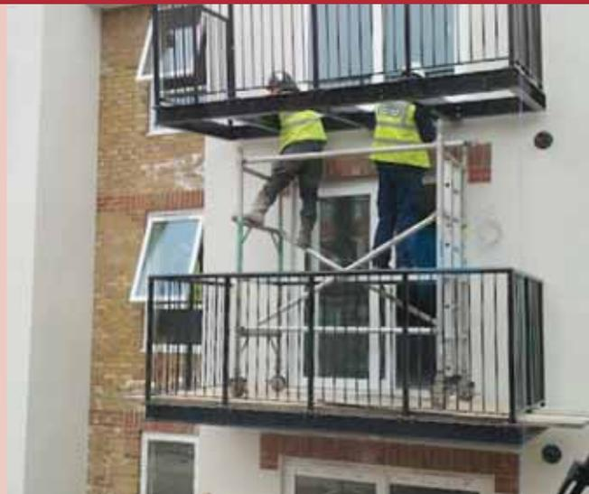
In this example from Dartford in Kent, we have an inadequate guardrail - a diagonal brace that does not fit and supported on planks - totally inadequate. But at least they have hi-vis vests and hard hats! Mistaken priorities?
