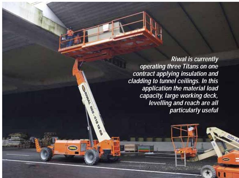
*Rival is currently operating three Titans on one contract applying insulation and cladding to tunnel ceilings. In this application the material load capacity, large working deck, levelling and reach are all particularly useful*
