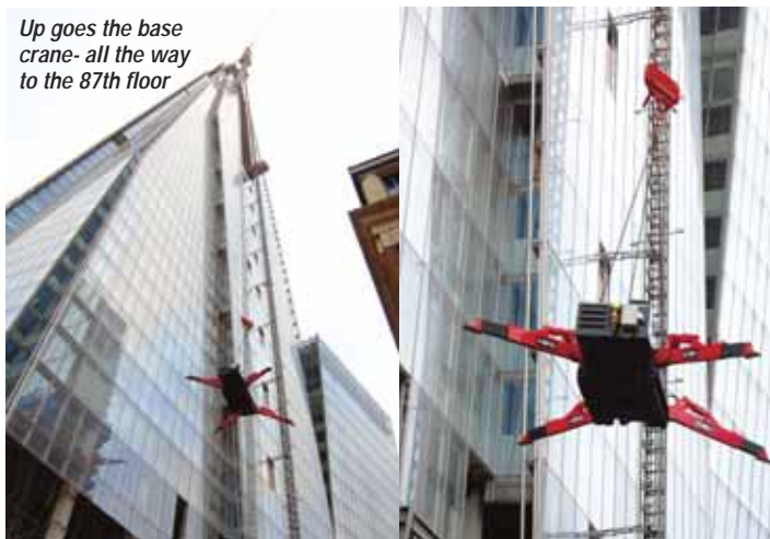
Then the boom is reinstalled
