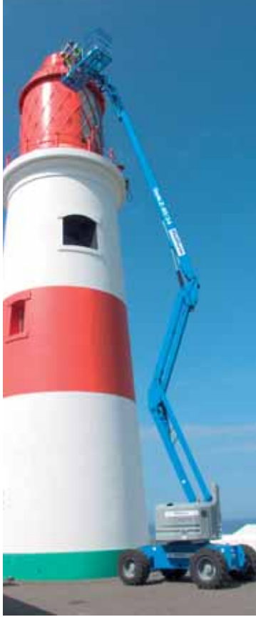
The Platform Company supplied a Genie Z60/34 articulated boom to carry out work on the Souter lighthouse
