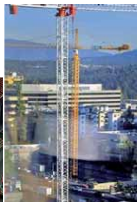
(Above) A picture taken prior to the collapse shows the crane (rear) was possibly up to a metre off vertical.
