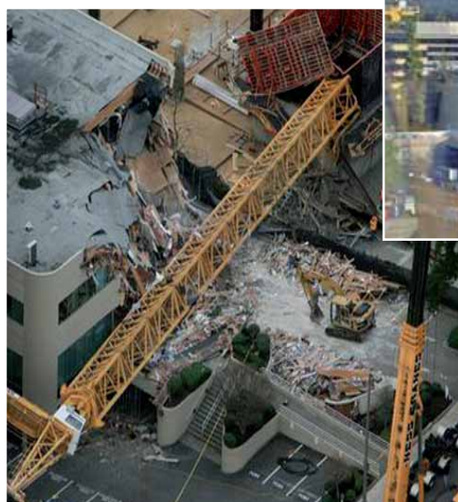
When the foundation of the crane failed it caused massive levels of damage killing a man in a top floor apartment. The crane driver survived.
