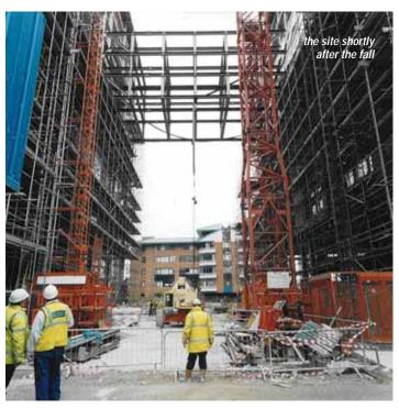
He was standing on scaffolding and using a set of chain blocks to move a steel beam into place above him, when bolts holding the blocks in place gave way, causing them to fall on him. His hands became entangled in the chains which dragged him over the guardrail and 25 metres to his death.
