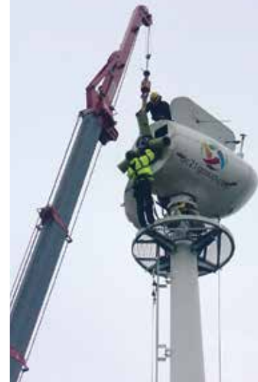
On top of the 25m tower
