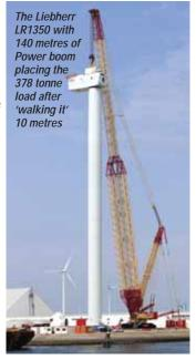
Norbert van Schaik, Repower's local site manager believes that this is one of the heaviest single wind turbine nacelles ever lifted onshore by one crane, as in most cases the drive train is lifted individually, or components are only fitted once the housing has been placed.
