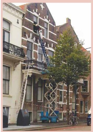
A man in Vlissingen, the Netherlands combines his ladder with a 20ft narrow aisle scissor to reach a window. When the photographer explained the risks of overturning the scissor by his make do methods he responded that he was being very careful!
