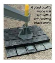
suitability. The problem with such material is that some timber will split easily when under load. While the use of a number of lengths of wood, requires a level of expertise to set up safely, so that it does not move or kick out from under the outrigger jack. Differing timber thicknesses complicates the task still further.
