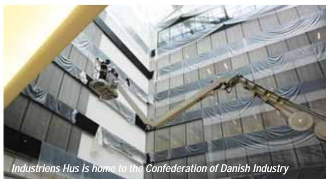
The Falcon FS320 is being used for maintenance work on the Industriens Hus building
