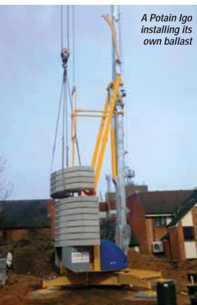
Self-erectors can set up in the most unusual and remote areas
