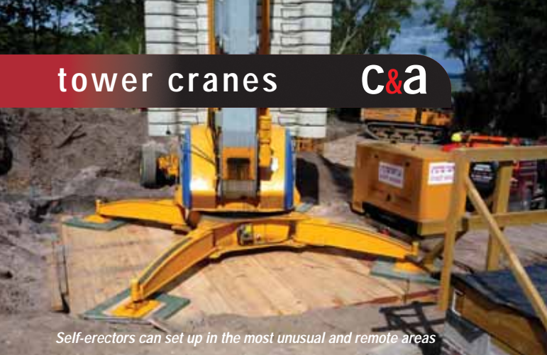
A Potain Igo installing its own ballast
