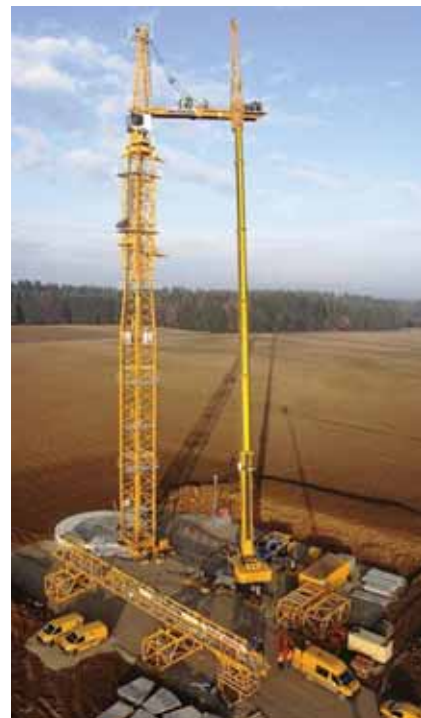
One of the main advantages of using a tower crane is the reduced amount of space needed to erect the crane.
