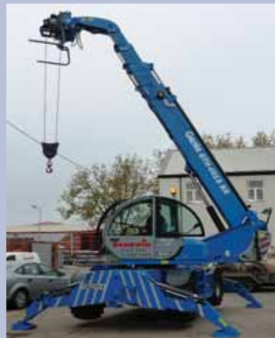
The telehandler is used to unloaded components, carry lift and position them ready for fixing at a height of 17 metres.
