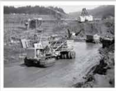
May Photo - A Cat RD4 crawler and No. 22 pull grader at work. Weighing 3,575 pounds and wielding an eight-foot blade, the No. 22 was produced from 1936 through 1942, the year that Cat discontinued all pull graders. (Caterpillar, Inc. image, HCEA Archives)
