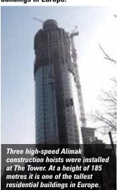
Two of the hoists - the 100 metres a minute, 3,200kg capacity Scando 650 FC-S 100 - are specifically designed to speed up construction time and save costs with a full height transit time reduced to just 90 seconds, compared to more than four minutes using standard hoists. The hoists also incorporate VFC drives which have improved levelling accuracy and power savings of around 30 percent.
