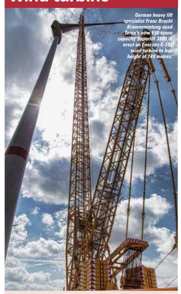
Developed with lifting large wind turbines in mind German heavy lift specialist Franz Bracht Kranvermietung used Terex's new 650 tonne capacity Superlift 3800 to erect an Enercon E-101 wind turbine to hub height of 149 metres. The Scharrel community wind farm at Saterland's Ostermoor bog in Germany is built with a focus on big wind turbines in order to generate "green" electrical power.
