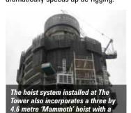
lift capacity of 5,500kg for the fast
