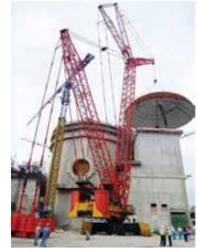
A Sany SCC9000 with 66m boom, 54m jib and 51m superlift radius to hoist the dome of No3 generating set which weighs 155t, is 11m high and 37m in diameter.
