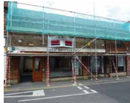
The Wantage scaffold
