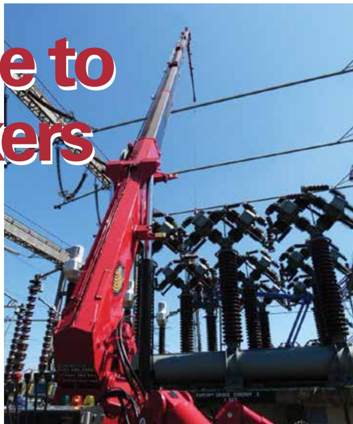
from an access platform making sure each silencer was slung securely. Working at an 11.5 metre radius, the crane removed all the 16 silencers, then made a return visit
