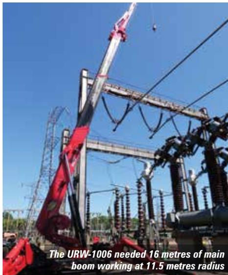
The URW-1006 needed 16 metres of main boom working at 11.5 metres radius
