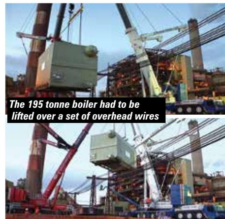
The 195 tonne boiler had to be lifted over a set of overhead wires
