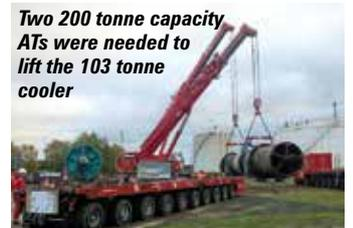
Two 200 tonne capacity ATs were needed to lift the 103 tonne cooler
