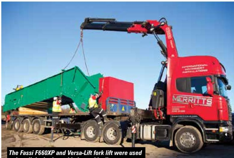
The Fassi F660XP and Versa-Lift fork lift were used to install the horizontal baler and incline conveyor
