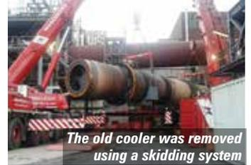
The old cooler was removed using a skidding system
