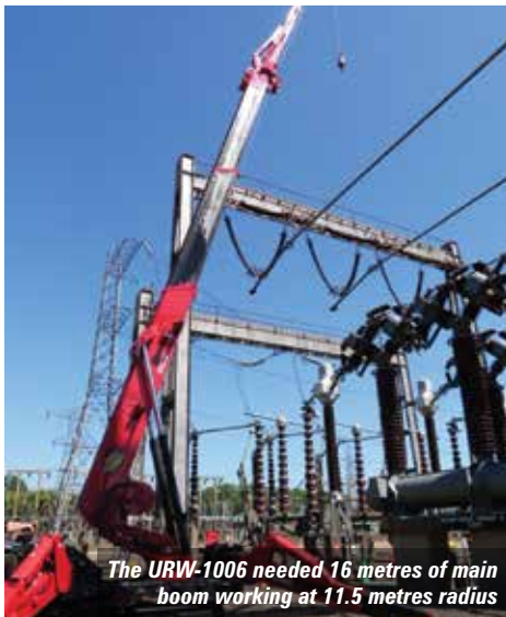
The 50kg silencers were lifted up and over the overhead power lines
