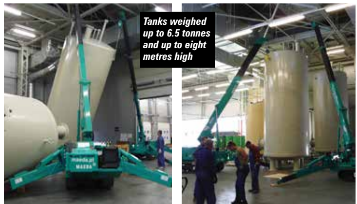
A slinger/signaller worked from an access platform making sure each silencer as slung securely
