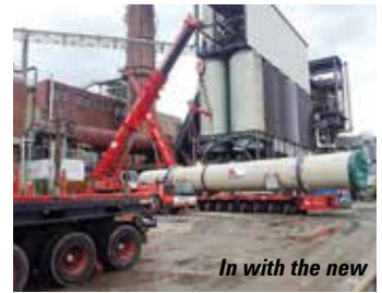
Two 200 tonne capacity ATs were needed to lift the 103 tonne cooler
