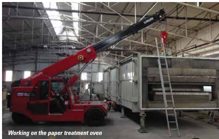
The F200E helping install seven tonne steel moulds in the injection moulding machine
